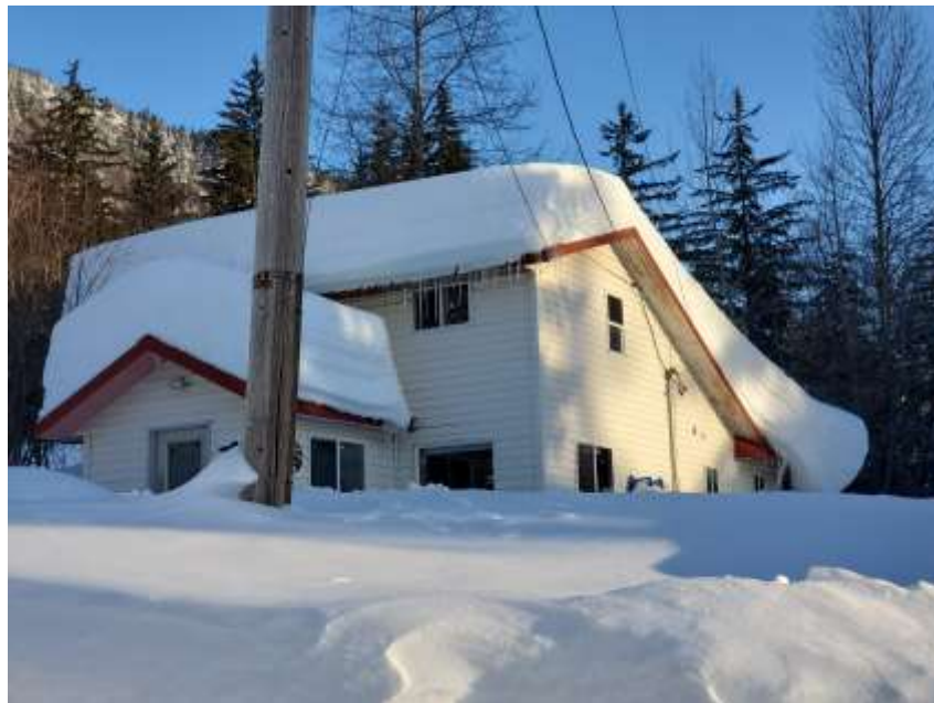
Caption: In January 2022, Haines was nearing record snow loading values on roofs that hadn't shed all winter. HAC began sounding the alarm on Social Media and assisting the public with assessing their roofs. Unfortunately, there were multiple roof collapses that occurred subsequently in Haines.
